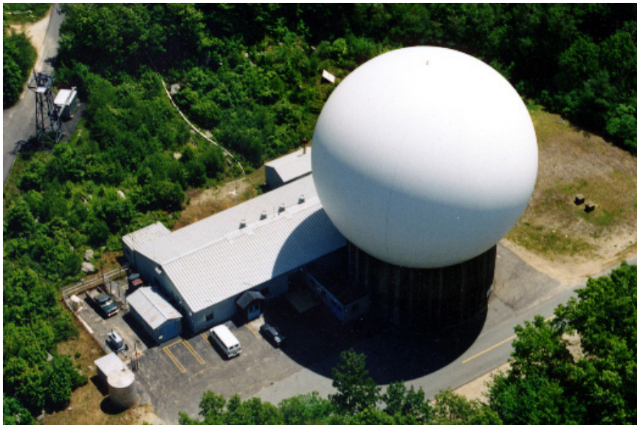
Figure 1. Aerial view of Westford site. The VLBI antenna is inside the radome. The WES2 GPS antenna is on top of the tower in the upper left corner of the photograph.
