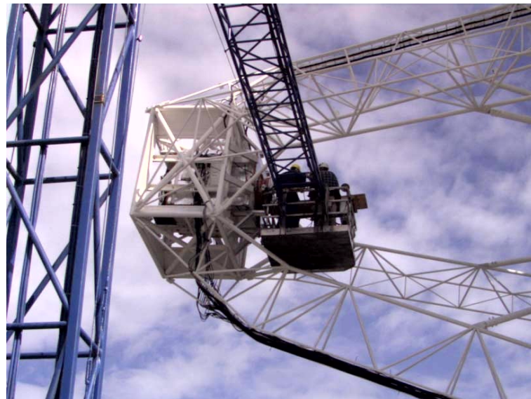
Figure 2. GCGO staff removing the receiver for dewar replacement
