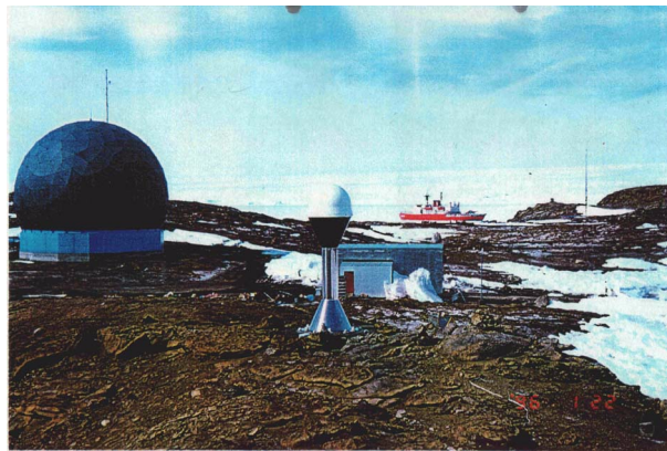
Figure 1. Syowa VLBI antenna with radome and the IGS GPS antenna
