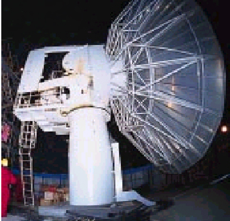
Figure 1. Because of weathering, about 20 radome panels were replaced with new ones in January 2002.
