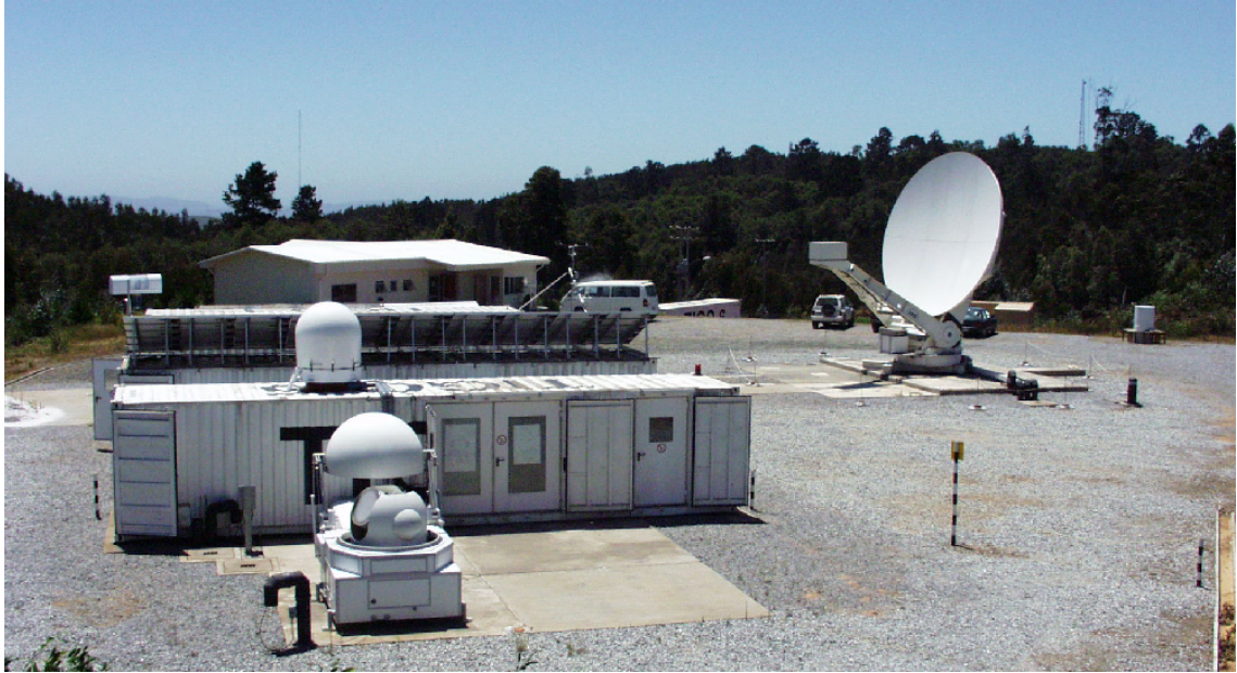
Figure 1. Geodetic Observatory TIGO: Instruments from left to right: water vapour radiometer, SLR Radar, SLR telescope, meteorological sensors, VLBI radiotelescope, local survey monument.
