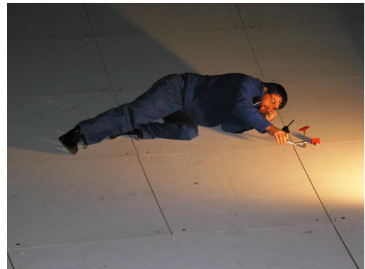
Figure 4. Jonathan Quick adjusts one of the mounting bolts.
