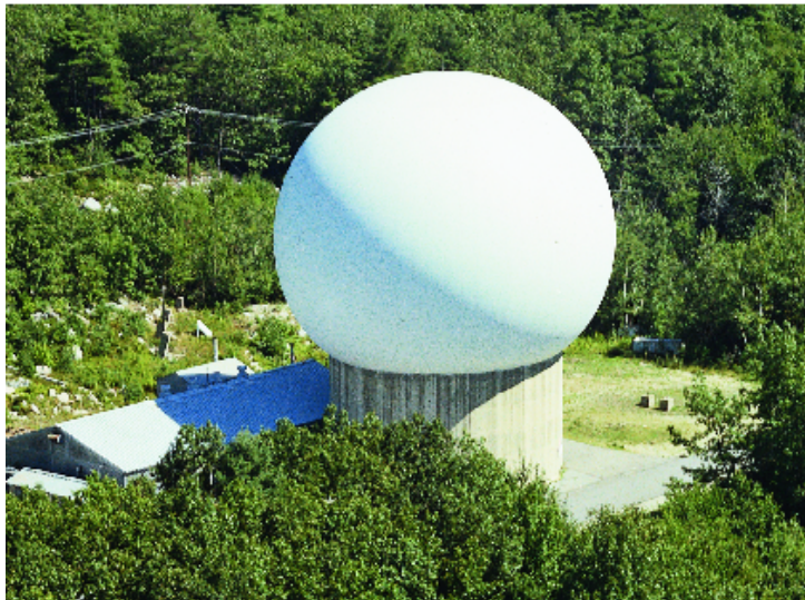
Figure 1. The radome of the Westford antenna.
