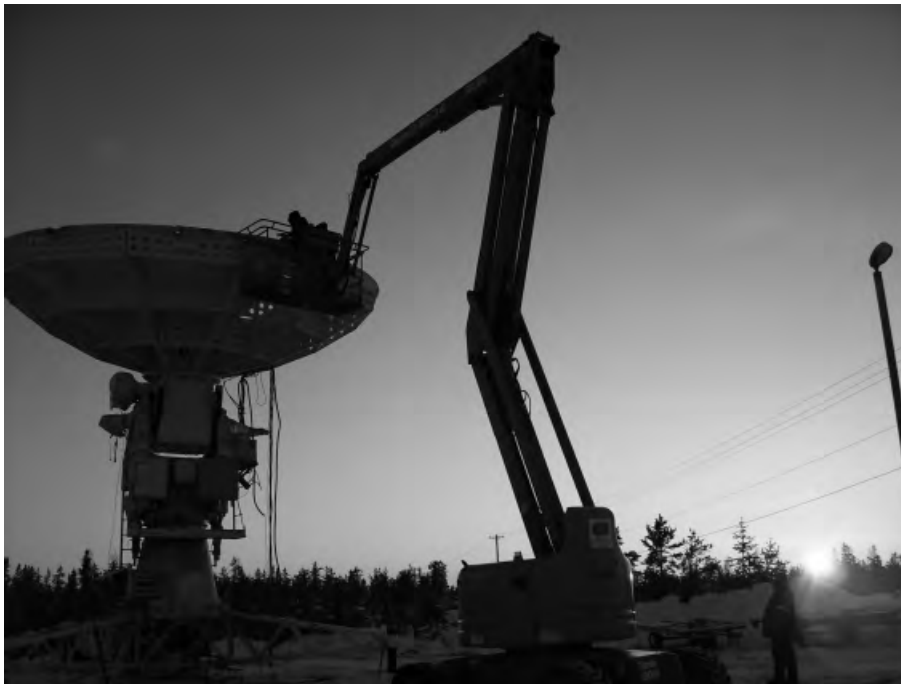
Figure 1. Dismantling the Yellowknife 9m antenna.
