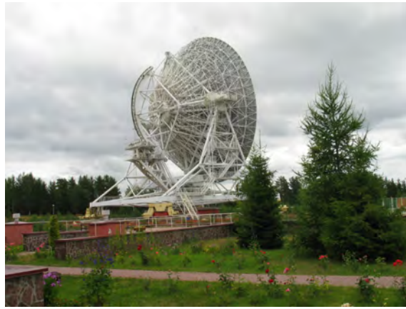
Figure 2. Current view of RT without large equipment cabin.
