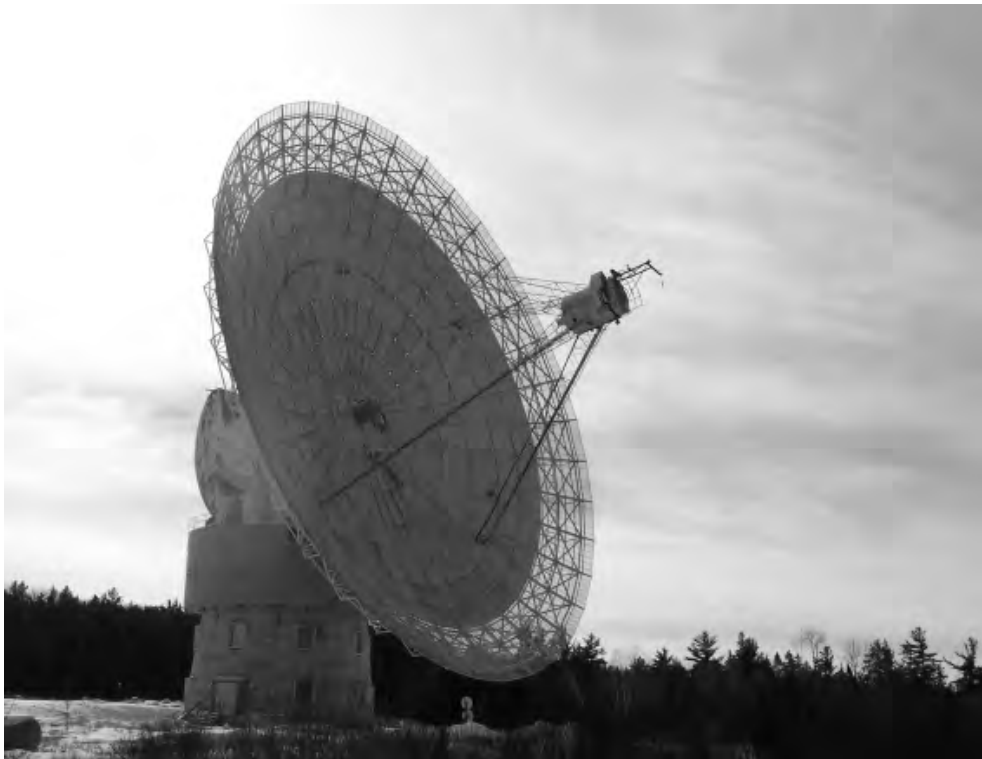
Figure 1. Algonquin Radio Observatory rests in its final position after 40 years of use.
