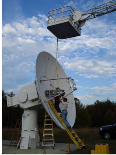
Figure 1. Jay Redmond and Bruce Whittier installing the Dewar on the 5 m MV-3 antenna.
