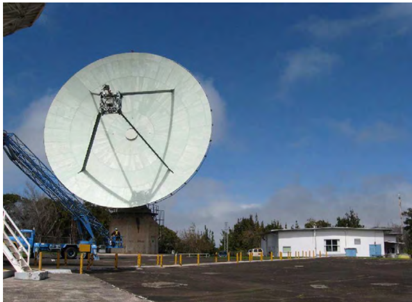
Figure 1. KPGO 20m antenna and operations building.
