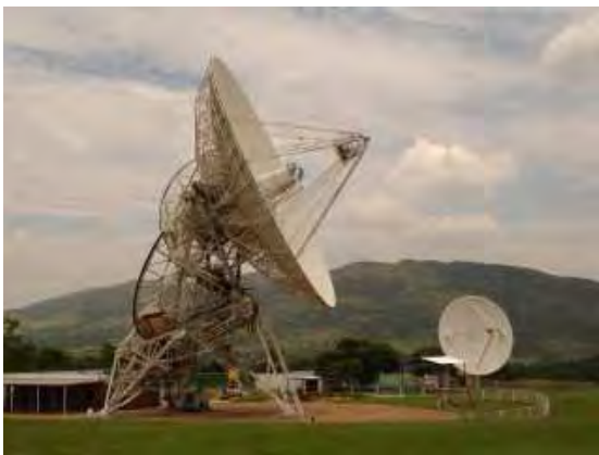
Figure 1. The 26-m HartRAO radio telescope with the 15-m XDM in the background. The XDM is a testbed prototype for the Karoo Array Telescope (KAT), which, in turn, will be used to test technology leading up to development of the Square Kilometer Array (SKA).
