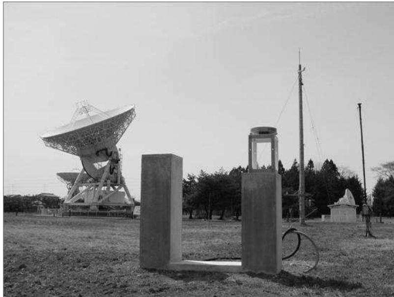
Figure 5. The Mizusawa GPS station under construction in 2006.
