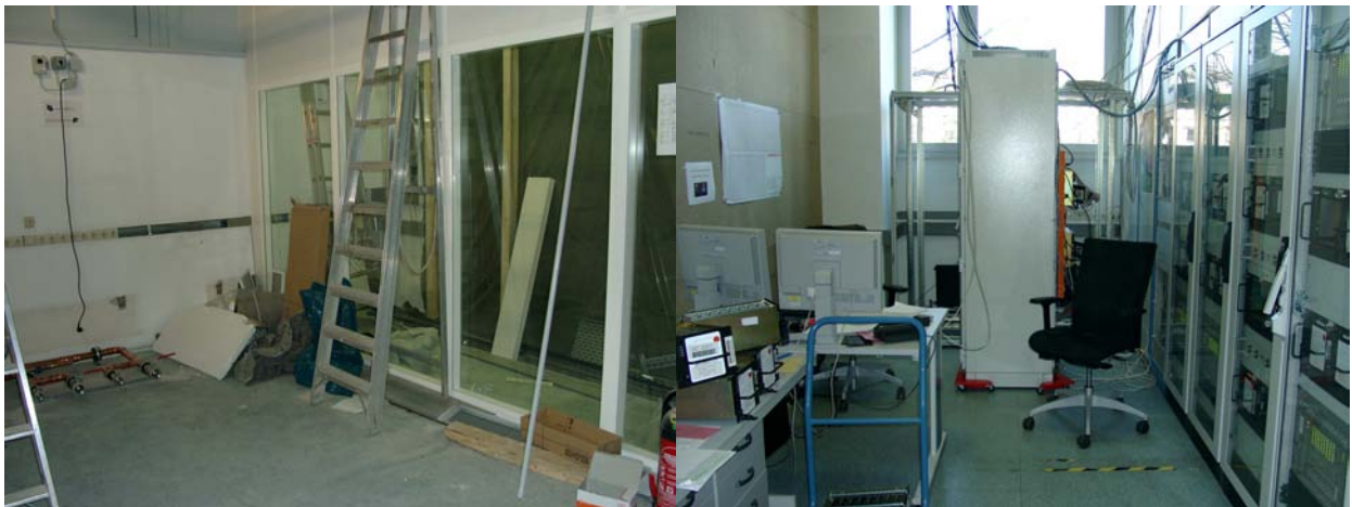
Figure 1. Left picture: sound and thermal insulation room for the software correlator still under construction, right panel: temporary correlator room with one Mark 5A rack (center - side view) standing in-room without cooling.
