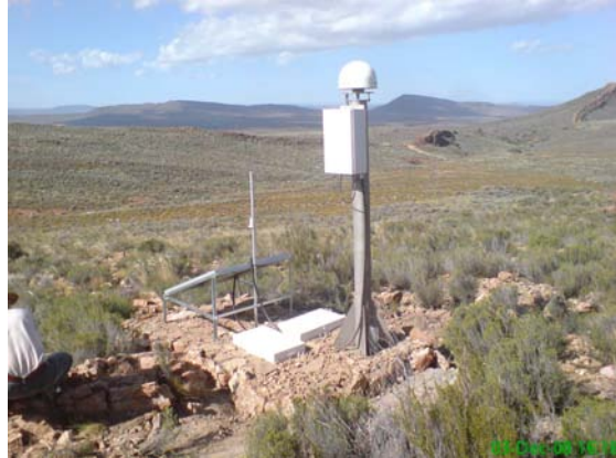
Figure 4. The new GPS reference station at the Matjiesfontein site.
