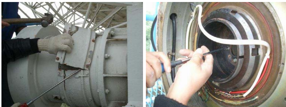
Figure 2. Fastening the elevation encoder screw in December 2008.
