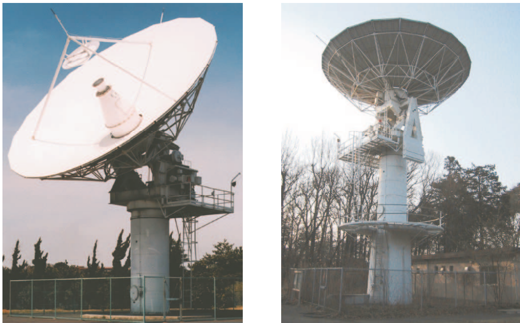
Figure 1. 11-m VLBI antennas at Kashima (left) and Koganei (right).
