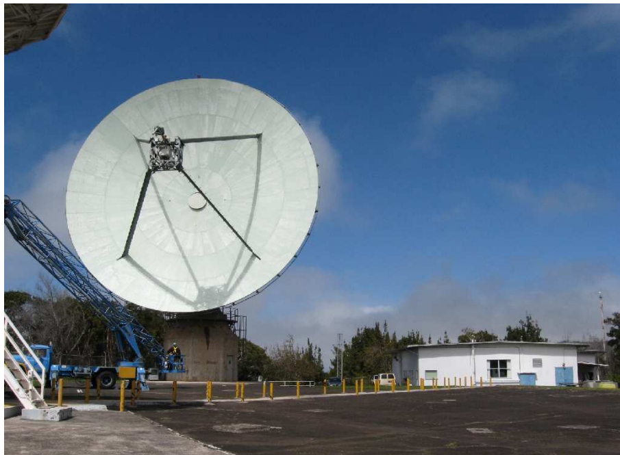
Figure 1. KPGO 20 m and operations building.
