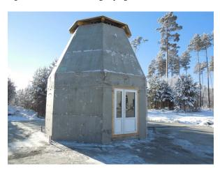
Fig. 5 Antenna tower for 13.2-m dish.
