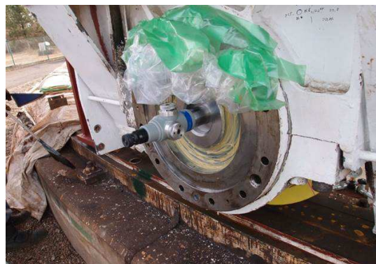
Fig. 2 Installation work of new azimuth wheel.
