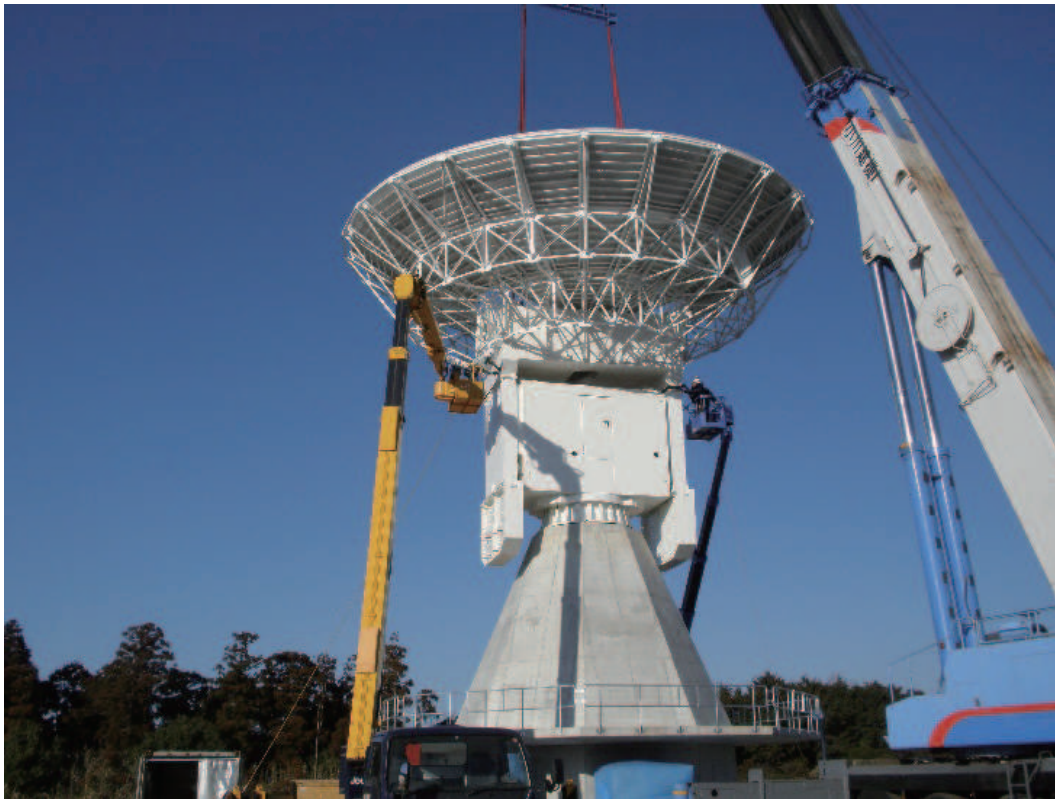
Fig. 5 Construction of the antenna.
