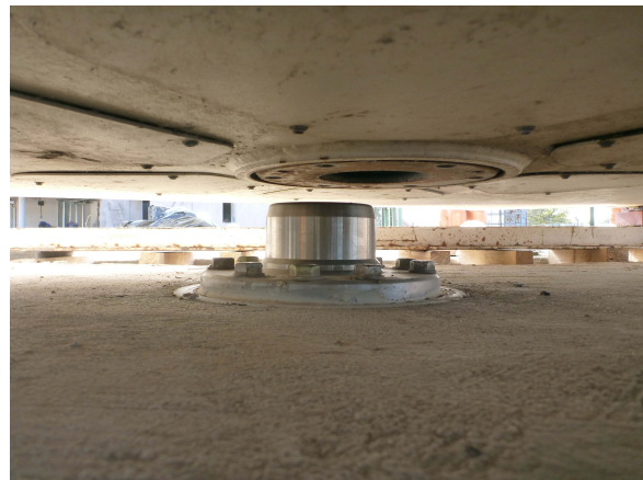
Fig. 4 The geodetic reference marker of the radio telescope is part of the platform. The radio telescope is centered above the marker, which is conical and self-centers the radio telescope during the setup (May 6, 2015). The acronyms used for this radio telescope reference marker are listed in Table 1.
