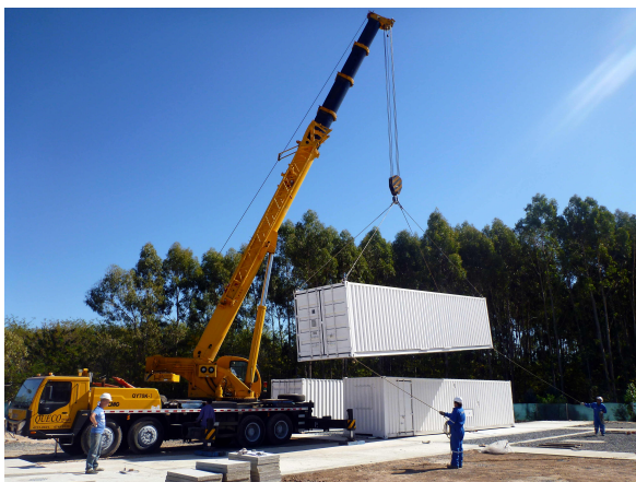
Fig. 2 Downloading the 23-t container with the radio telescope inside at the AGGO platform (April 20, 2015).
