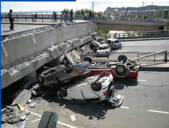
(top) The protective unreinforced concrete pipe of the GPS/Glonass monument of the IGS station CONZ was destroyed in the megaquake. The reinforced concrete pillar itself, however, survived the event without damage. (below) Collapsed component of a bridge crossing the Biobío river in Concepción with crashed vehicles.
