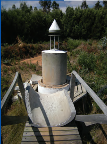
(top) The protective unreinforced concrete pipe of the GPS/Glonass monument of the IGS station CONZ was destroyed in the megaquake. The reinforced concrete pillar itself, however, survived the event without damage. (below) Collapsed component of a bridge crossing the Biobío river in Concepción with crashed vehicles.
