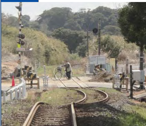
Twisted railway tracks near Kashima (Photo by T. Kondo).
