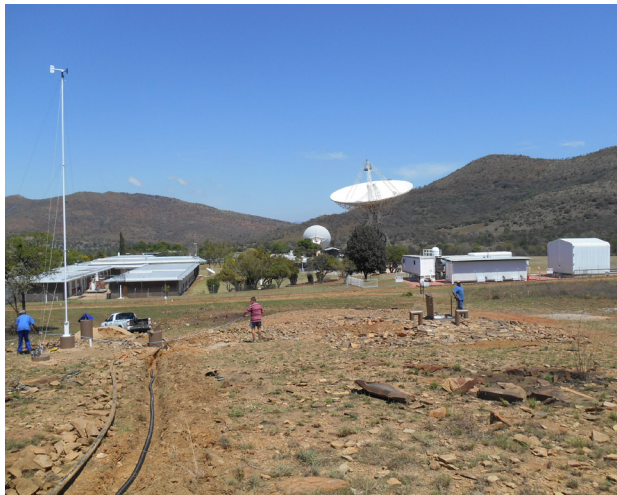
View of the current HartRAO instrumentation. The VGOS antenna will be installed towards the right of the photo, in line with the SLR to minimize RFI as SLR tracking is minimal in the north-south line.
