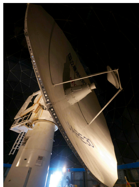
View of the Syowa site in winter with the radio telescope protected inside the radome.
