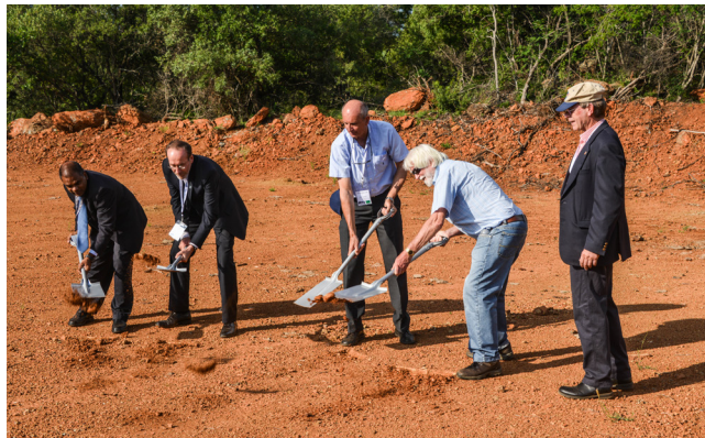
Groundbreaking for HartRAO's future VGOS telescope.
