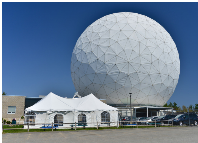
Main building of MIT Haystack Observatory with the radome of the 37-m antenna and the typical coffee/lunch break tent in the front.
