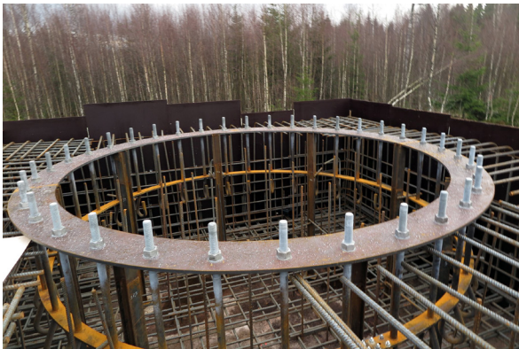
Base of the new radio telescope at Metsähovi before casting the concrete. Iron bars are firmly attached on the bedrock.
