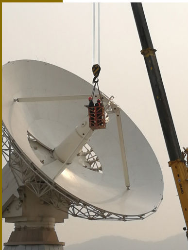
Workers are being lifted during the construction phase.
