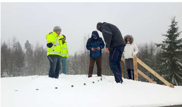
Base of the new radio telescope at Metsähovi before casting the concrete. Iron bars are firmly attached on the bedrock.
