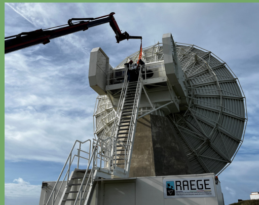
Installing the VGOS receiver on the radio telescope.
