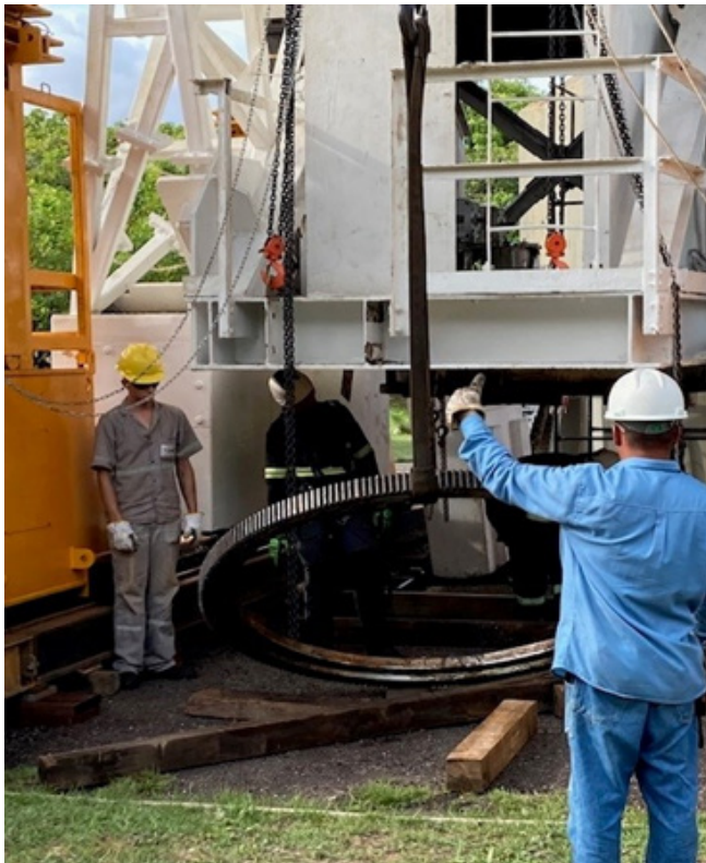
Removing the Damaged Azimuth Bearing.
