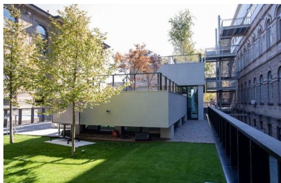
Fig. 1 Politecnico di Milano Campus Leonardo, new building 3A with three green roofs, where the PMD AC is hosted.
