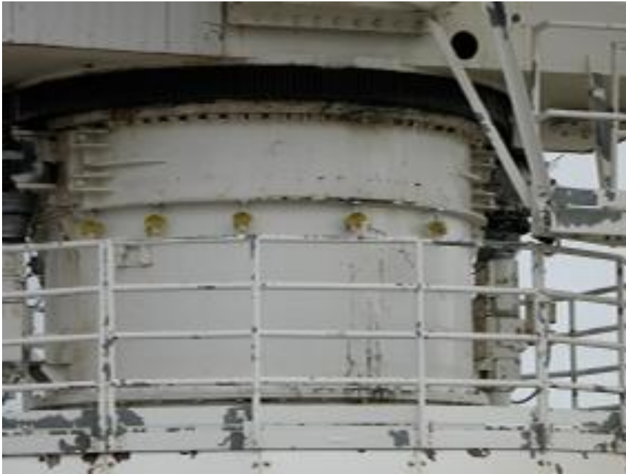
Prisms T1, T2, T3, T4, T5 at the telescope tower (not moving).
