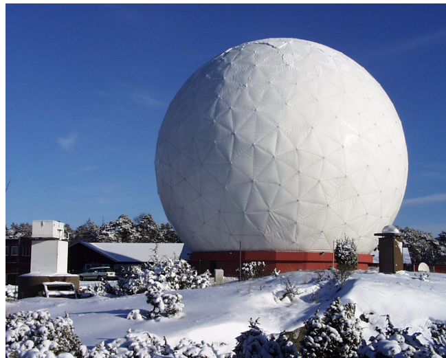
Figure 2: The 20 m radio telescope at Onsala enclosed inside the radome. Note the Onsala water vapor radiometer (WVR) and the GPS antenna of the Onsala IGS permanent station on the left hand and right hand side, respectively.
