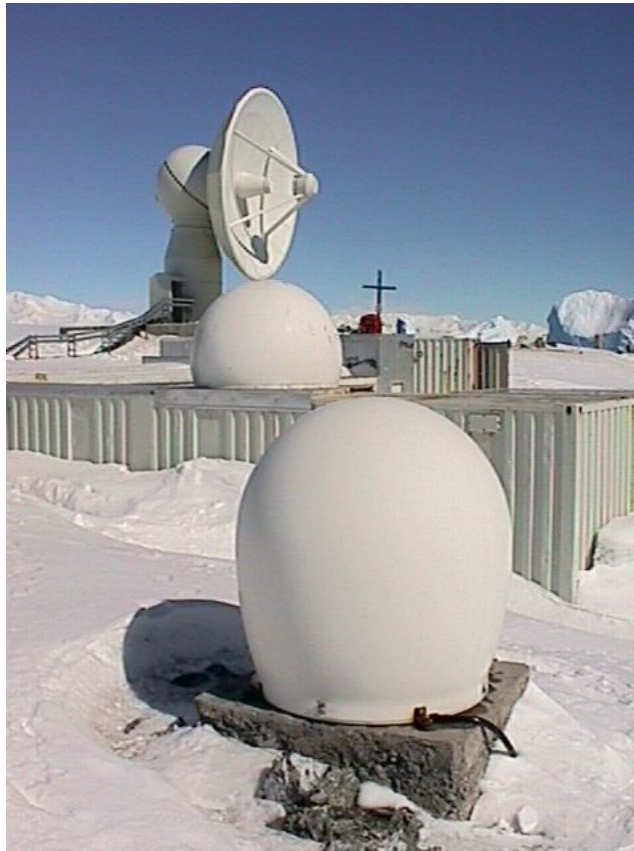
Figure 2. The VLBI Antenna at O'Higgins, in front the GPS-Antenna and the PRARE ground unit protected by different radomes (October 1999).
