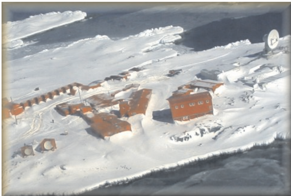
Figure 1. Geodetic Observatory O'Higgins - Antarctica: Air view to the German Antarctic Receiving Station (GARS) on the right hand and the Chilean Military Base on the left hand (picture taken at end of October 2002).
