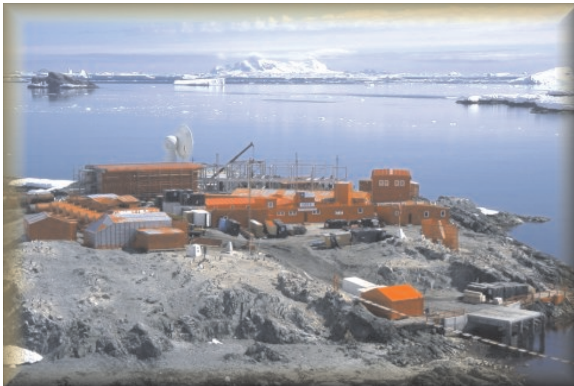
Figure 3. Geodetic Observatory O'Higgins - Antarctica: View from Rancagua mountain to the Chilean Military Base with the new constructed three-storied building. The GARS Station is hidden behind the building, only the antenna is visible (picture taken at middle of January 2003).
