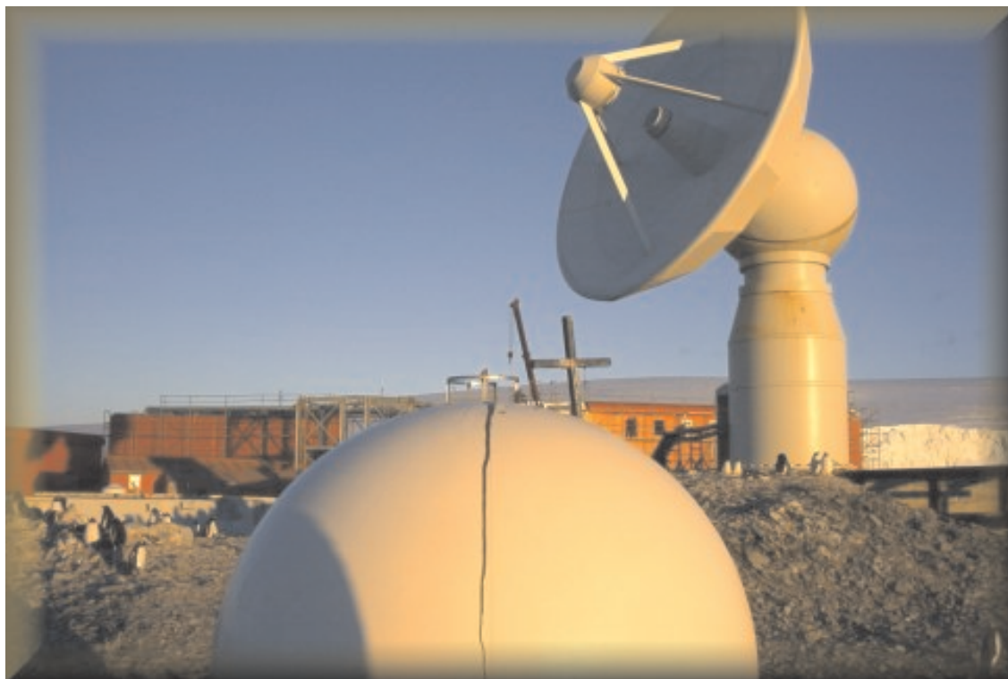
Figure 2. Geodetic Observatory O'Higgins - Antarctica: Horizon view of shifted Turbo rogue antenna in the direction of the new construction at the Chilean military base.
