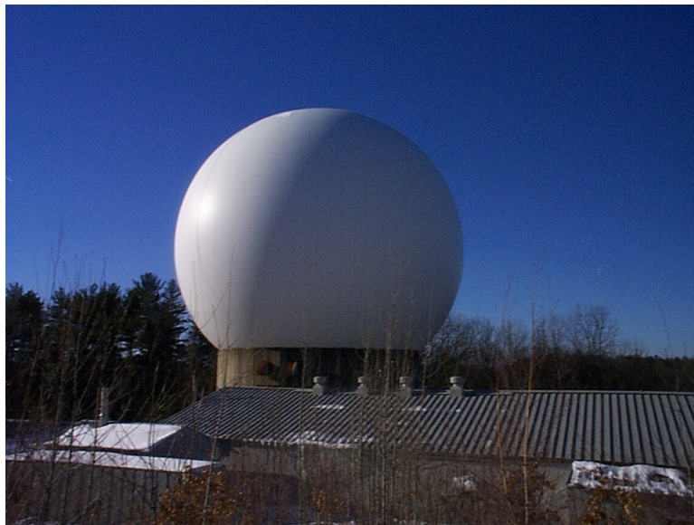
Figure 1. The radome of the Westford antenna.
