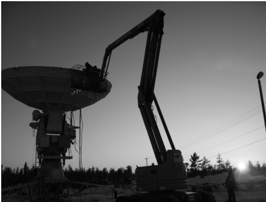
Figure 1. Dismantling the Yellowknife 9m antenna.
