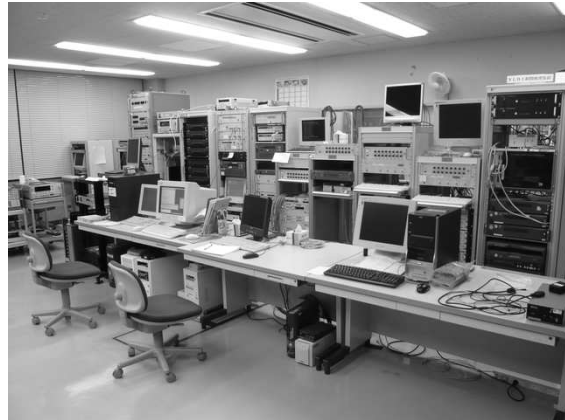
Figure 1. A view of the observation room of the Kashima 34m antenna. The K5 system in this room is used both for observation and correlation processing.
