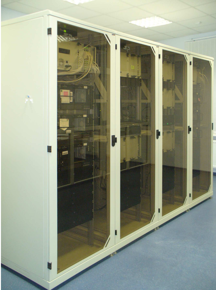
Figure 1. The 6-station IAA RAS correlator.
