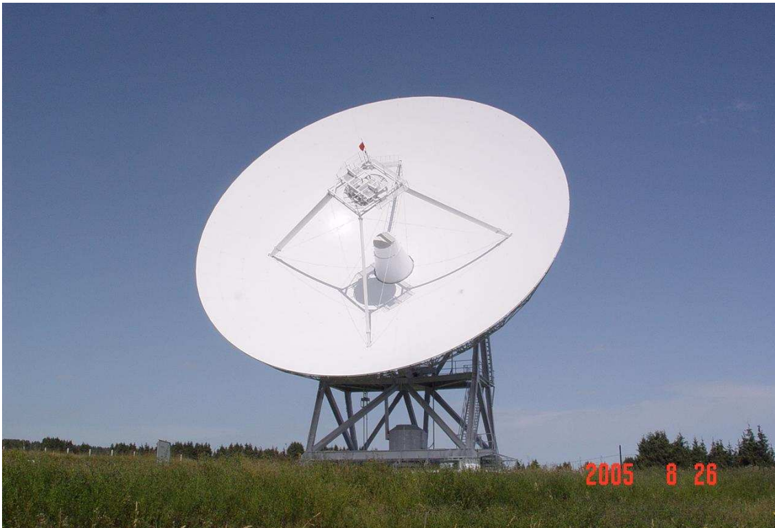
Figure 2. The 25-m, modified Cassegrain radio telescope of Urumqi Observatory was built in 1993.
