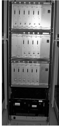
Figure 3. R1002M DAS and Mark 5B+ in Svetloe observatory.
