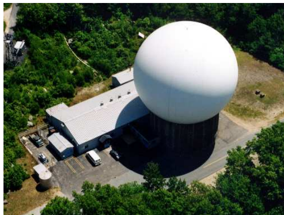
Fig. 1 Aerial view of the radome and facilities of the Westford antenna. (For scale the diameter of the radome is 28 m.)
