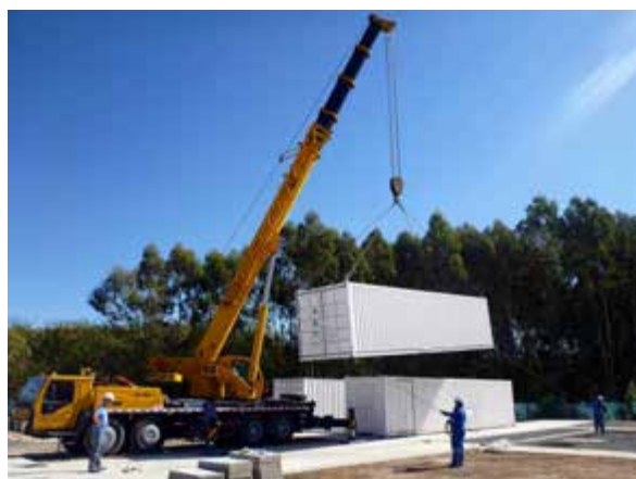
Fig. 2 Downloading the 23-t container with the radio telescope inside at the AGGO platform (April 20, 2015).
