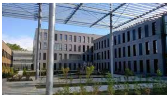
Fig. 1 The new OASU building that has hosted the LAB and the Bordeaux IVS Analysis Center on the Campus of the University of Bordeaux in Pessac since June 2016.
