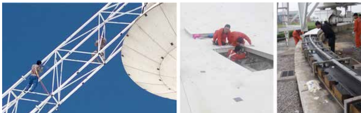
Fig. 2 Antenna maintenance of the Tianma 65-m telescope.
