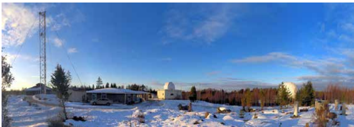
Fig. 1 A view of the Metsähovi Fundamental Geodetic Station. At the center of the picture is the new building of the SLR telescope. At right, the radome of the 13.7-m radio telescope of Aalto University can be seen.
