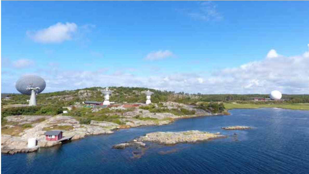
Fig. 3 The Onsala telescope cluster in 2016 with the new Onsala Twin Telescopes in the center of the photo. The new VGOS radio telescopes are equipped with reflectors of 13.2-m diameter. The radio telescope on the left hand side is the 25.6-m telescope installed in 1964, which is the first European telescope ever to be involved in VLBI. First geodetic VLBI measurements were performed already in 1968. The white radome on the right side of the picture houses the 20-m radio telescope installed in 1976, which was used with the Mark III geodetic VLBI system since 1979 and has the longest time series in the International VLBI Service for Geodesy and Astrometry (IVS) database. Close to the radome, but not visible in the photo, is the GNSS station ONSA, which was established already 1987 in the CIGNET network, several years before the International GNSS Service (IGS) was founded. ONSA had a pioneering role in the early days of GNSS, and has the longest continuous time series in the IGS network. There is also a gravimeter laboratory with a superconducting gravimeter. Shown in the picture foreground is the Onsala super tide gauge inaugurated in 2015. The observatory is one of the unique fundamental space geodetic sites that have a direct access to the sea level and co-locate VLBI, GNSS, gravimetry, and sea level monitoring. It is thus an important co-location site for the Global Geodetic Observing System (GGOS).
