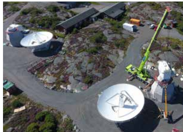
Fig. 1 Photo of the OTT taken on 15 August 2016 during the lift of the azimuth cabin on to the concrete tower of the northern telescope. The two reflectors and the azimuth cabin of the southern telescope are still on the ground. The telescope towers have no cladding yet.
