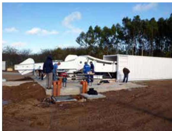
Fig. 3 The re-installation of the former TIGO radio telescope as AGGO radio telescope above a specially constructed platform was performed with the support of the company MT-Mecatronica from Chile (May 6, 2015).
