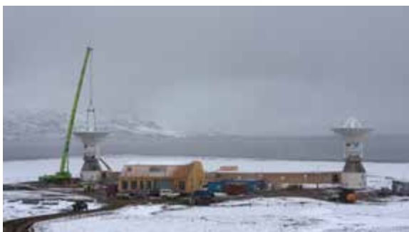
Fig. 6 Main reflector installation on the north telescope of the new observatory.
