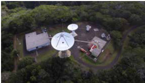
Fig. 2 KPGO site overview after installation of the 12-m, removal of the 9-m, and removal of the 7-m.
