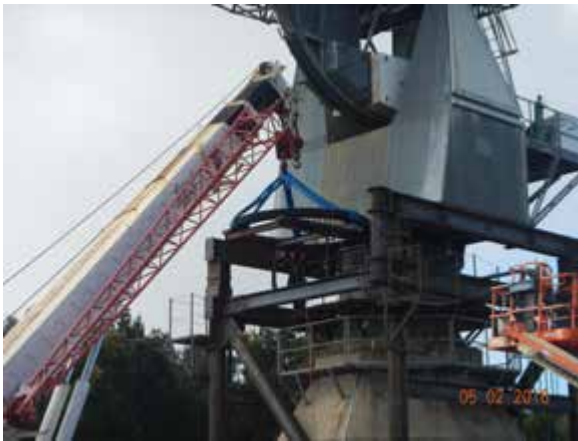
Fig. 3 20-m telescope azimuth bearing replacement effort.
