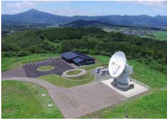
Fig. 2 Ishioka Geodetic Observing Station.
