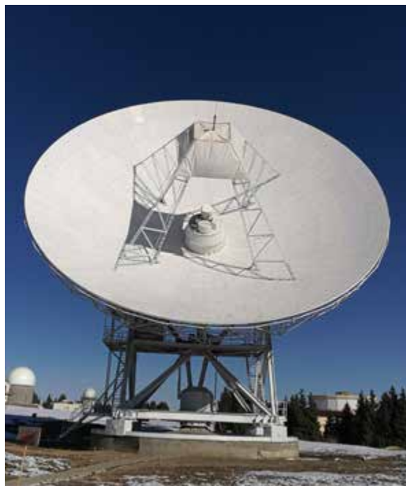
Fig. 1 The new NanShan 26-m Radio Telescope (NSRT).
