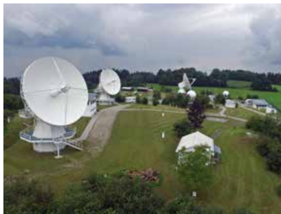
Fig. 5 The Wettzell triple of VLBI antennas: the Twin Telescope in the front and the 20-m telescope in the back (photo: Liu).
