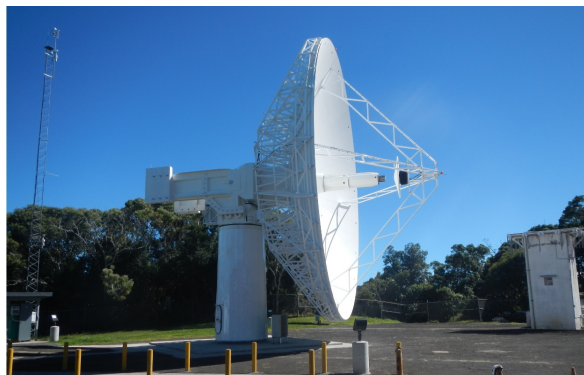
Fig. 1 Newly installed 12-m VGOS telescope at KPGO.
