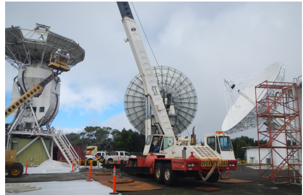
Fig. 4 9-m telescope demolition effort, with the 20-m and the 12-m operating in the background.
