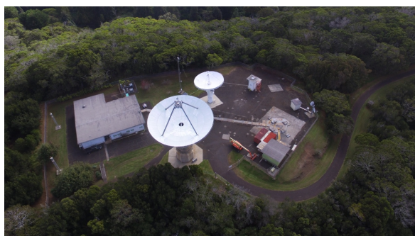
Fig. 2 KPGO site overview after installation of the 12-m, removal of the 9-m, and removal of the 7-m.
