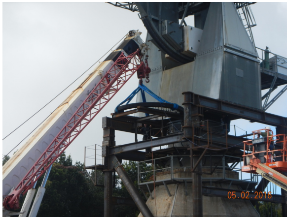
Fig. 3 20-m telescope azimuth bearing replacement effort.
