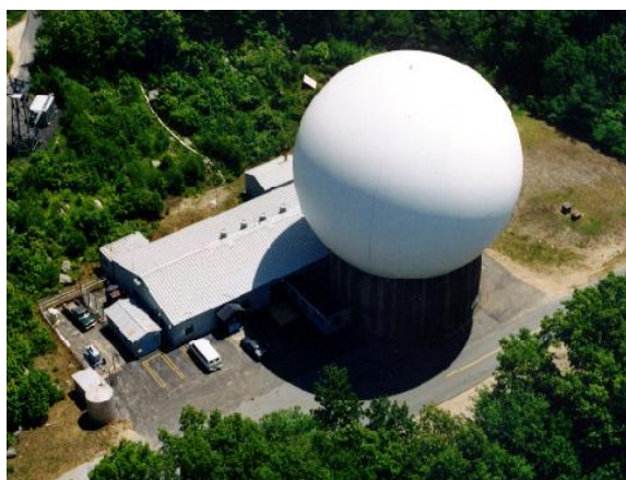
Fig. 1 Aerial view of the radome and facilities of the Westford antenna. (For scale the diameter of the radome is 28 m.)
