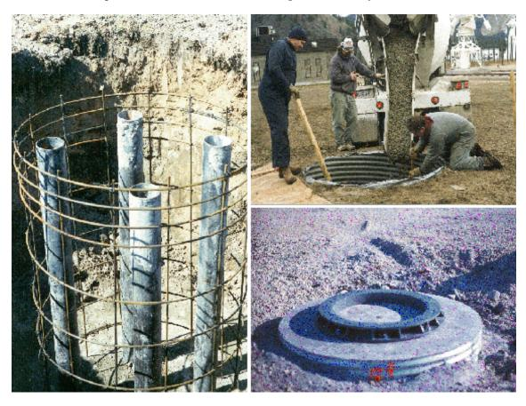
The concrete pad is anchored to be drock using 15 cm diameter steel well casing and 1 cm reinforcing steel bar. A transition ring is used to fix the antenna to the pad. It takes about 2 weeks to prepare the site and survey the local stability network.
