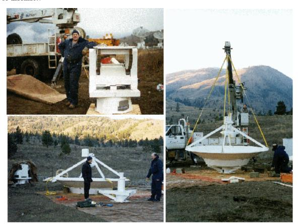
First, the two halves of the reflector, the quad legs, the sub-reflector and the S and X feeds are secured together on the ground. Second, the aluminum base is secured to the transition ring. Third, the positioner is secured to the base and levelled. Finally, the assembled dish is secured to the positioner.
