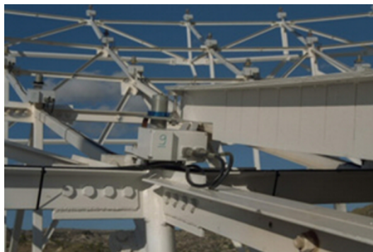
Figure 1. Actuators of the active surface installed in Noto.
