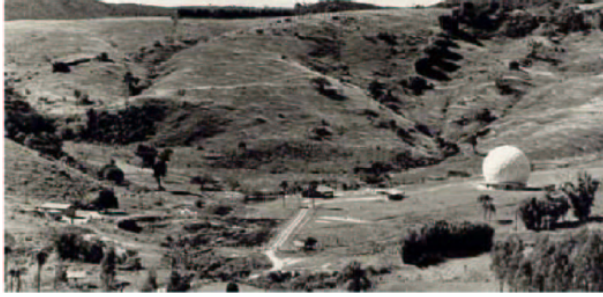
Figure 1. The Itapetinga Radio Observatory, Atibaia, near São Paulo city, with the 13.7-m radome-enclosed antenna built in 1971.
