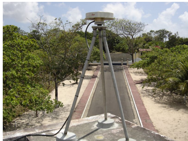
Figure 5. The new NOAA GPS antenna installed on the roof of the main ROEN building.
