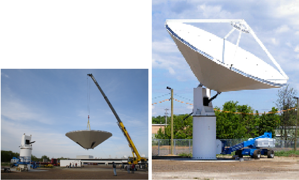
Figure 3. Constructing the 12m antenna.
