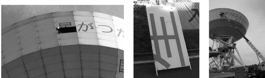
Figure 4. Tsukuba 32-m antenna repairing
