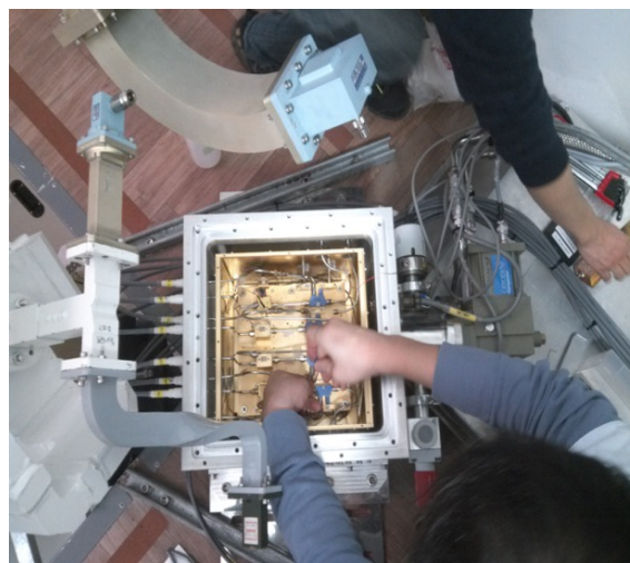
Fig. 4 LNA cooling chamber. Inside the chamber, LNAs for S/X, a cabling system for calibration, and mode switch cables (Hot/Cold/Sky) are installed.
