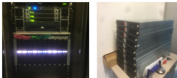
Fig. 5 Image of the computing cluster installed at the TWIN operations room with the spare nodes.
