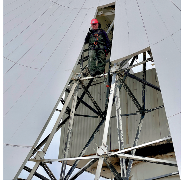
Fig. 4 The colleagues from Greenbank Observatory working on the 20-m antenna, taking panels from the parabola and gear boxes as spare parts.
