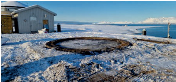
Fig. 7 The area where the 20-m antenna had been located, once the decommissioning was finished.
