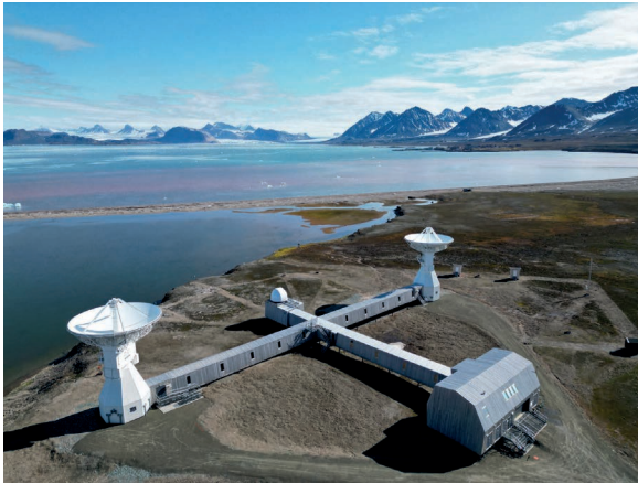
Fig. 2 The Ny-Ålesund geodetic observatory with the 13-m twin telescopes. From left to right: Ny-Ålesund 13-m North antenna (Nn) which is currently contributing in both the IVS VGOS and legacy networks, SLR dome, and Ny-Ålesund 13-m South antenna (Ns) which has been contributing in the IVS legacy network with parallel observations with the 20-m antenna (Ny). Operations building on the right front.
