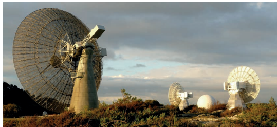
Fig. 1 VLBI radio telescopes operated at the Onsala Space Observatory: the 25-m (left) and the radome-enclosed 20-m legacy telescopes, as well as two 13.2-m VGOS antennas.
